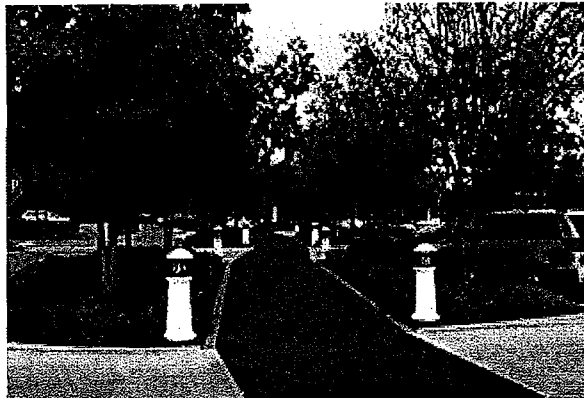
Bollard Lighting Example
