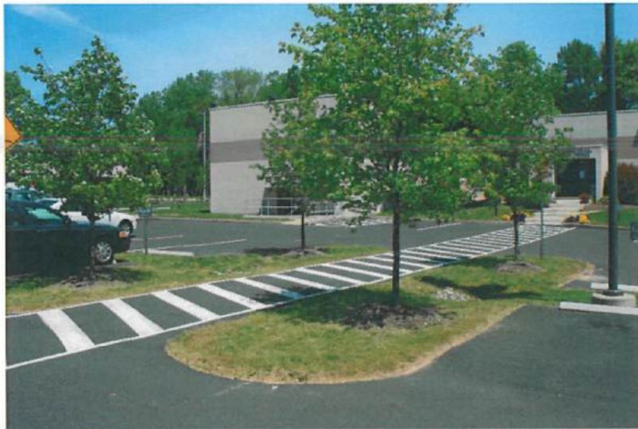
Walkways across parking aisles and through or adjacent to planting strips make parking lots safer and more accessible
