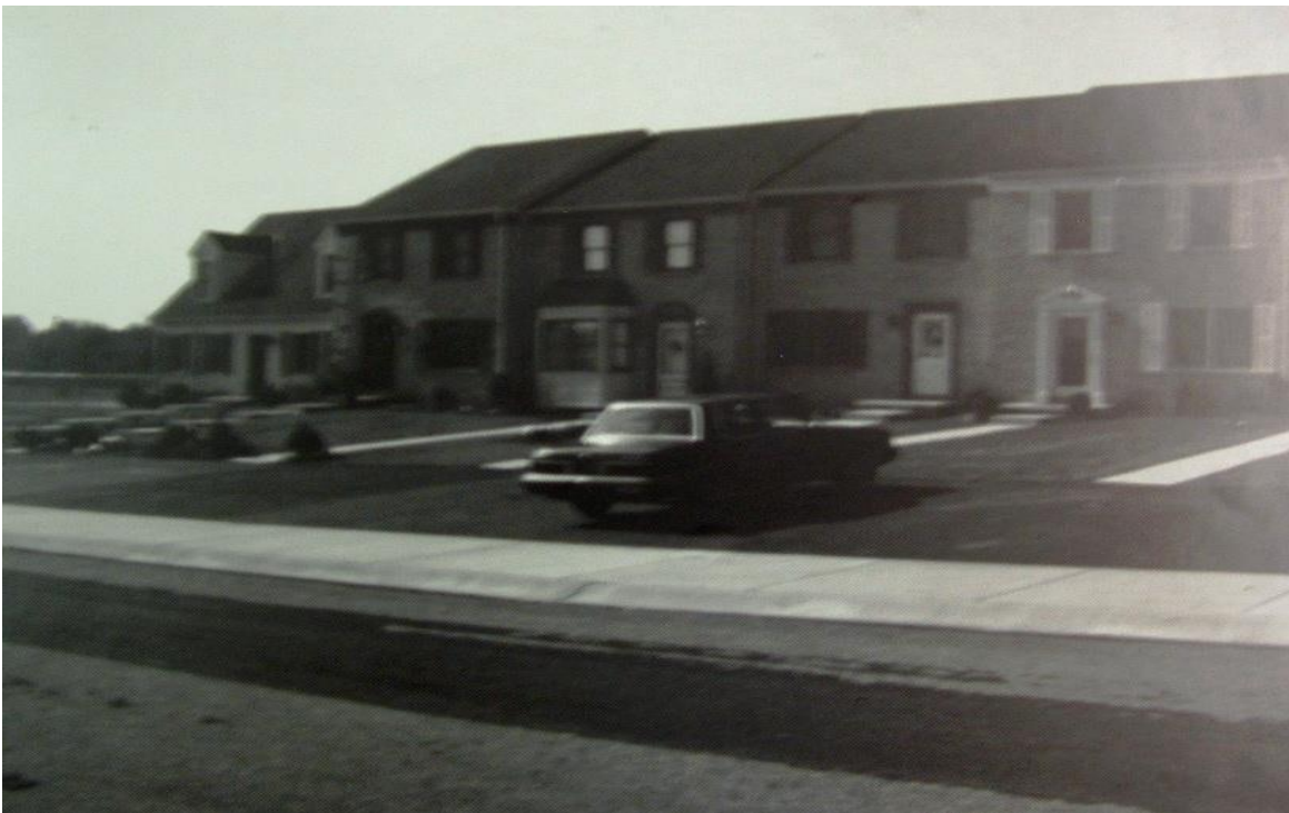
Illustration 9 — Multifamily residential development in Manheim Township with a negative VPS rating.
