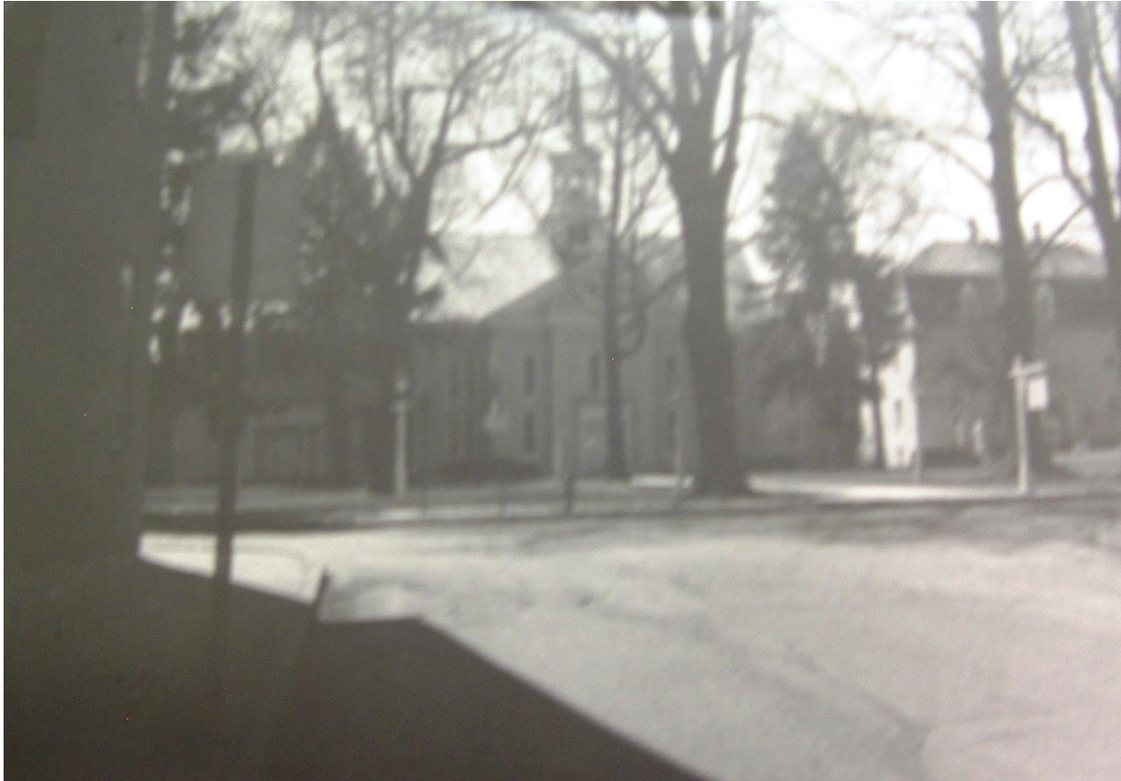
Illustration 53 — Buildings for public and semipublic uses, community clubs and community facilities should be prominent by virtue of additional mass and height, civic architectural design, or other distinguished features.
