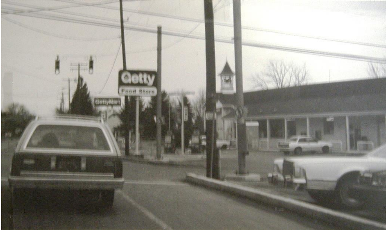
Illustration 5 — Commercial development in Manheim Township with a negative VPS rating.
