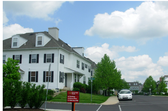
Larger Manor House, Lantern Hill TND.
