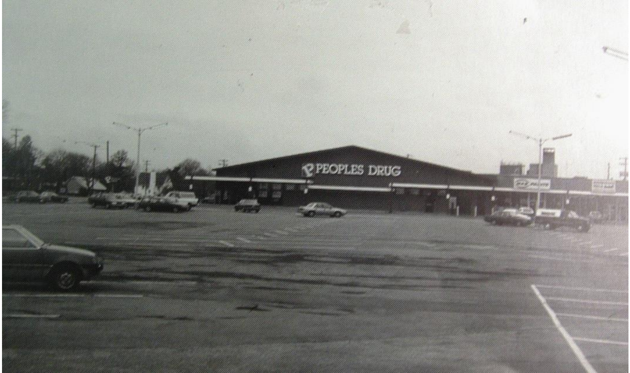
Illustration 3 — Commercial development in Manheim Township with a negative VPS rating.
