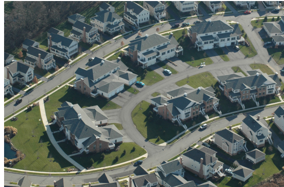
Attached units surrounded by single-family detached and semi-detached dwellings, Weatherstone TND.
