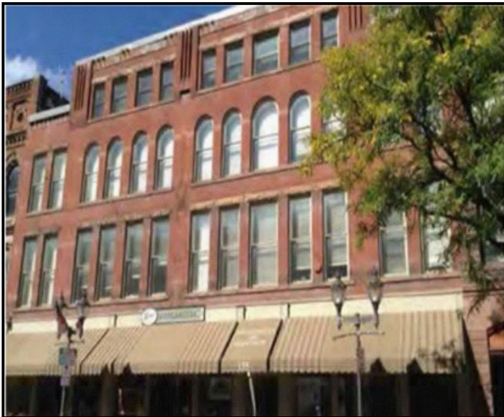
Figure 2. Windows, doors and architectural articulation shall be uniform and shall be regularly centered.
