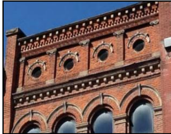
Figure 1. Example of Top Floor Cornice and Parapet.
