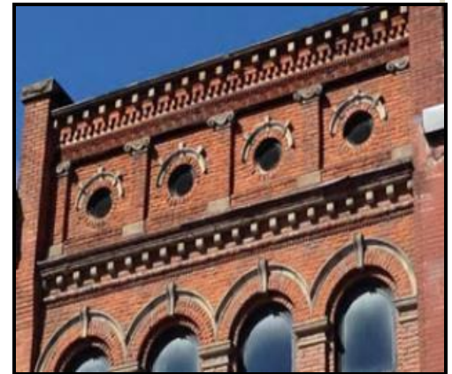
Figure 4. Decorative Parapet 153 Main St.
