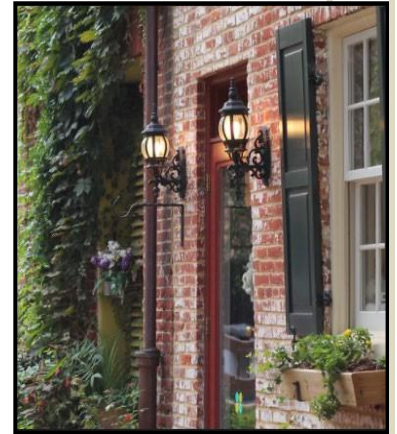
Figure 6 Main entrance luminaires
