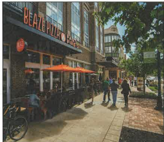
Figure 5.2: Street with paver furniture zone along the back of curb
