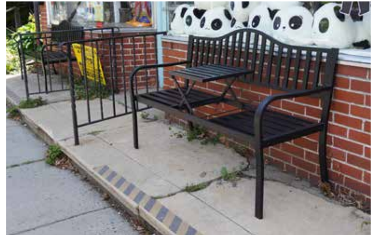
Unique benches with a pull-out tabletop are offered outside of this Main Street business, but the step is a barrier to accessibility.
