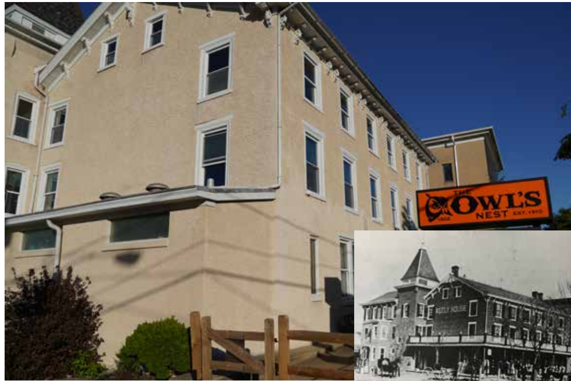
Although the former Keely House has seen many alterations throughout its long history, the building has retained its original window openings.
