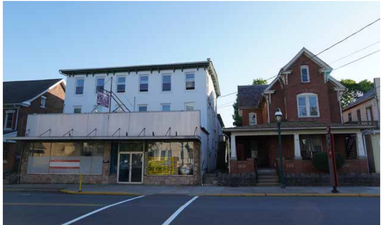
Examples of an unaltered front porch (right) and an addition or potentially enclosed porch (left)
