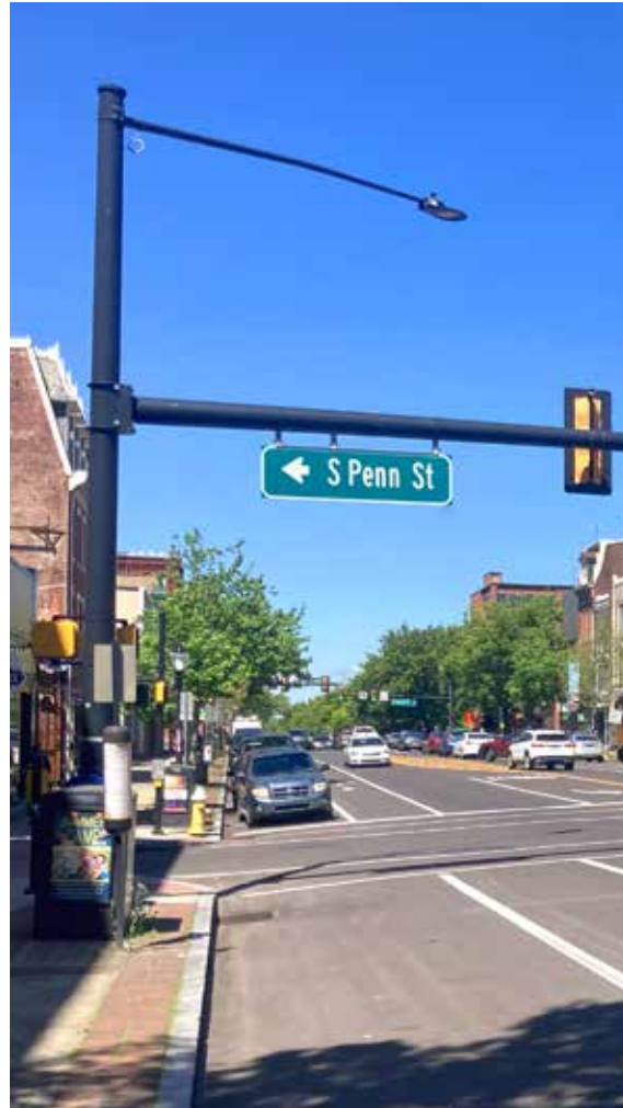
A black, decorative traffic signal pole and support arm in Pottstown Borough
