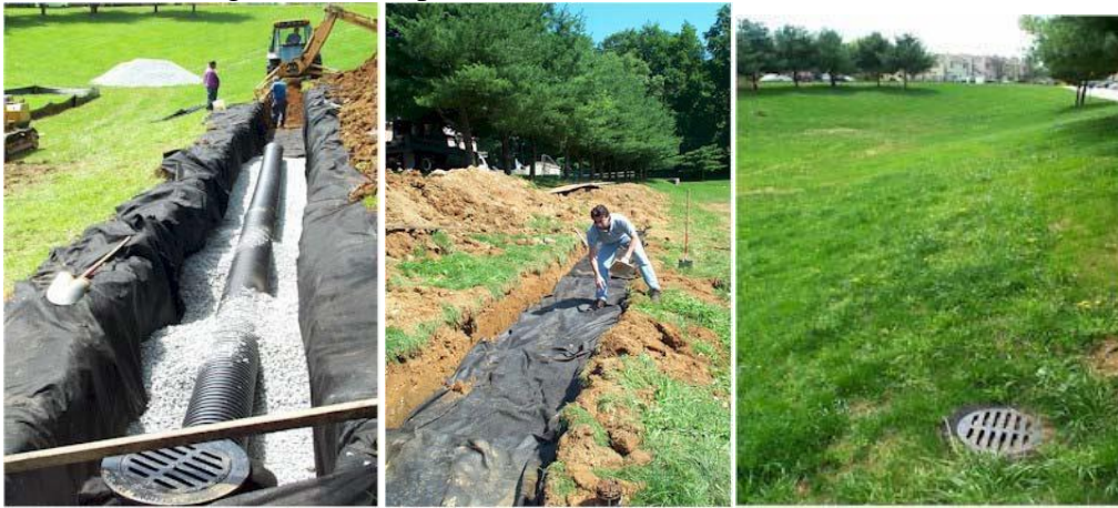
Figure 3: Example of Infiltration Trench Installation
