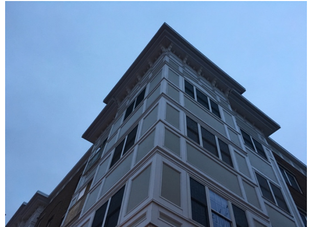
Picture 3 – Example of a deep cornice with exterior millwork and decorative paneling on the facade
