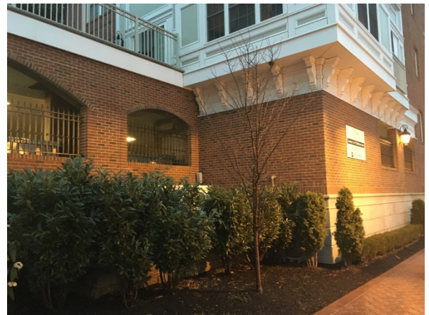
Picture 5 – Example of a decorative treatment for a parking garage opening and decorative millwork
