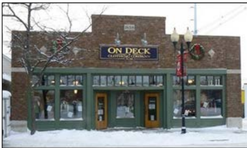
Figure 11.23. Second Highest-Rated Image for Commercial Signage.
